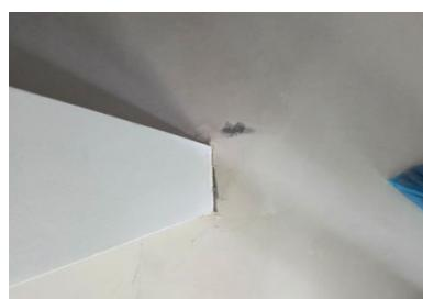
➔ **Tip:** Color-adapted substrate preparation, e.g. a light leveling compound for light LOBA StyleColor shades or a dark leveling compound for dark shades, makes minor workmanship imperfections due to insufficient layer thickness more forgiving..
