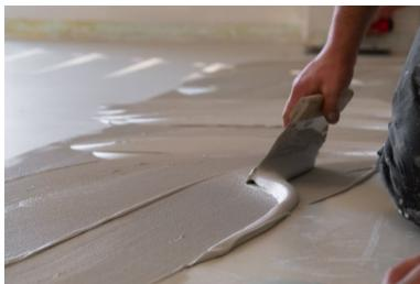
→ **Tip:** **Check the trowel blade regularly.** Worn notches can reduce layer thickness and lead to color deviations or insufficient coverage.
